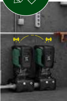
One piece of a traditional booster set with two pumps
